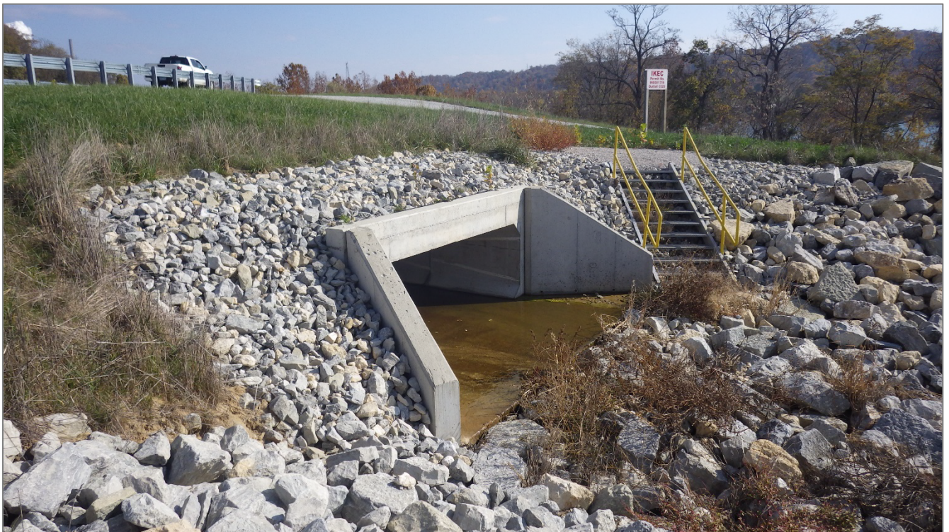
Photograph 12 – Downstream side of dam at 12 ft. x 4 ft. culvert.
