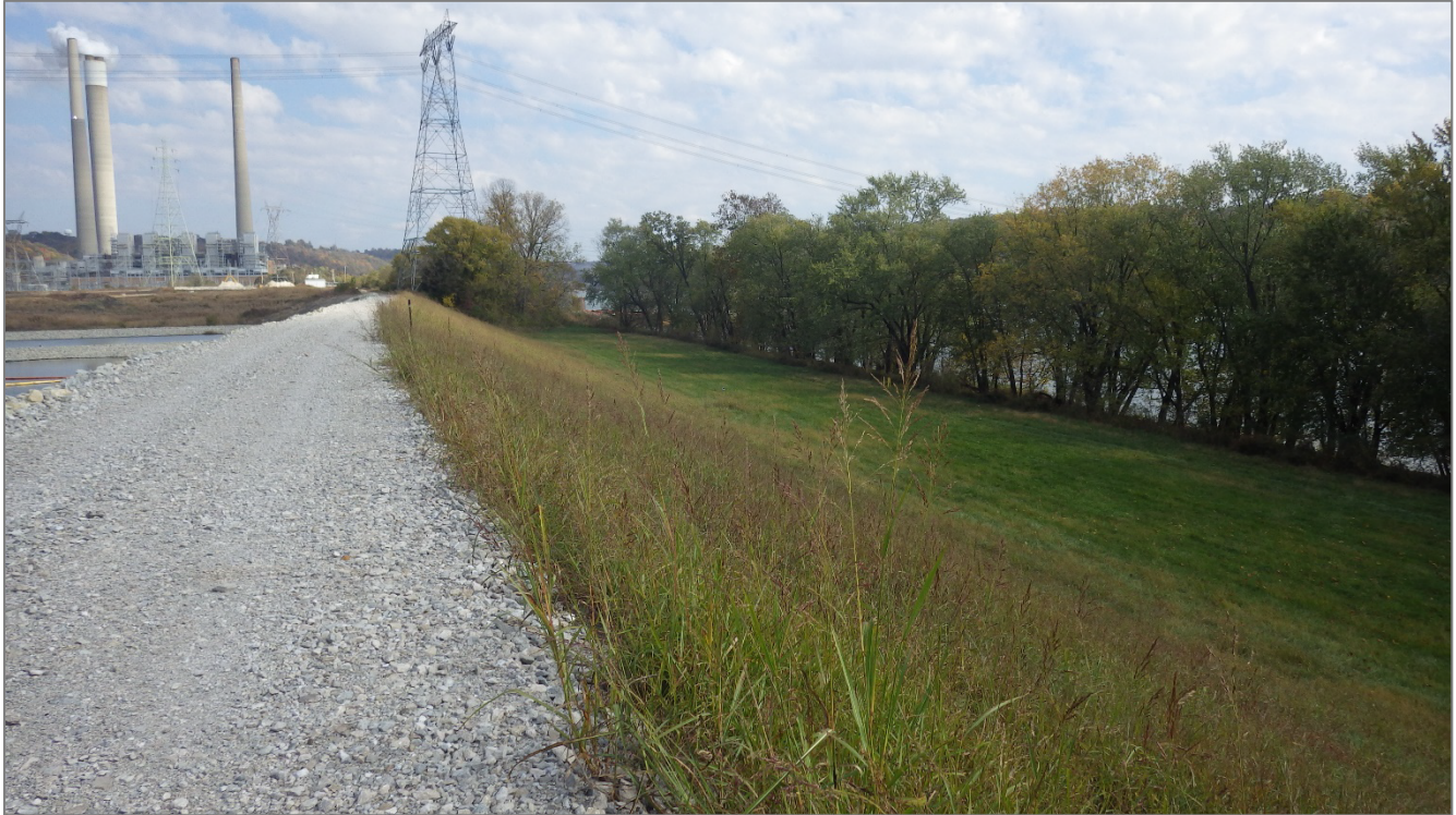
Photograph 3 – Exterior southwest dike embankment, looking east.
