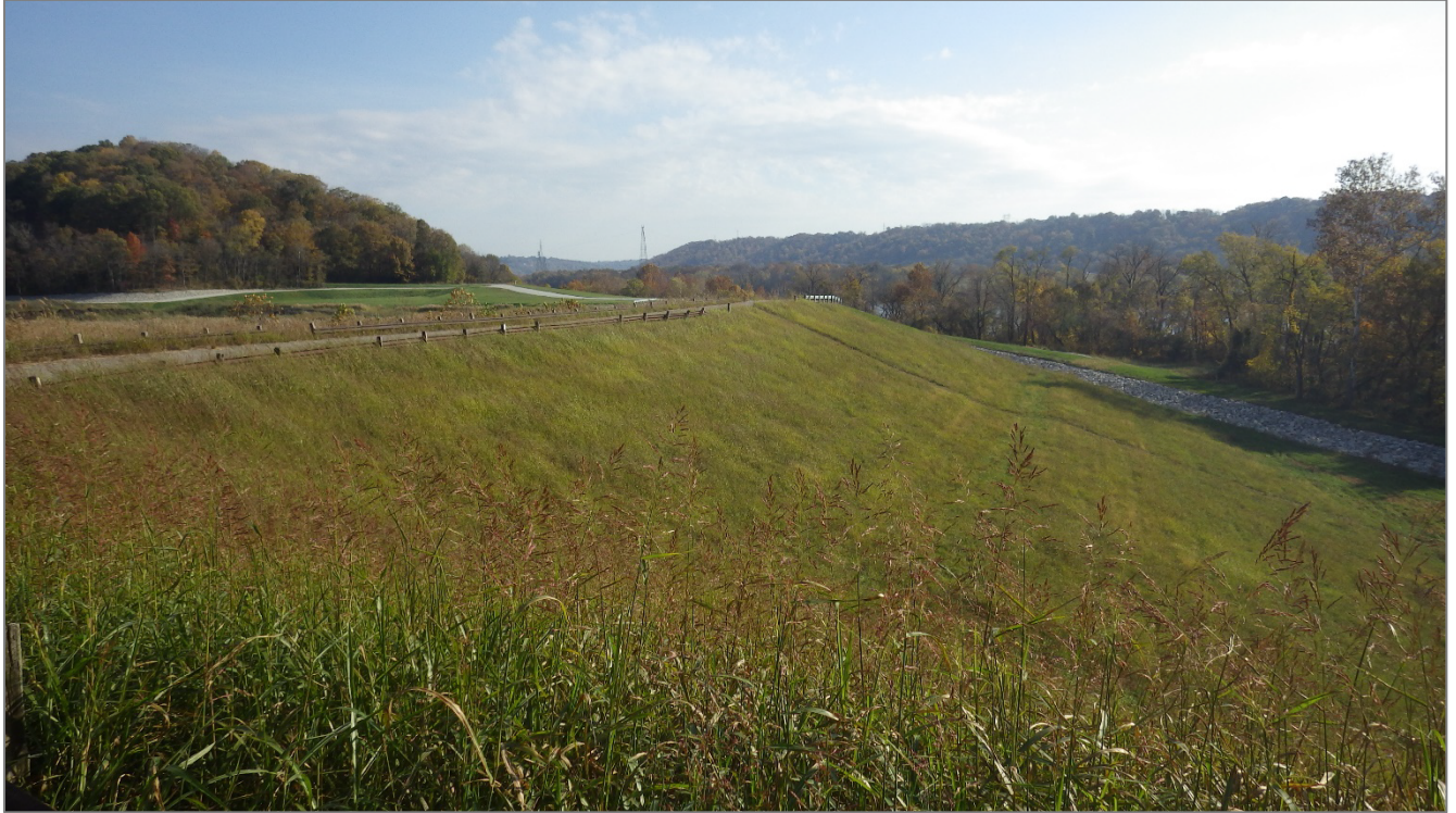
Photograph 1 – West downstream side of LRCP looking east.
