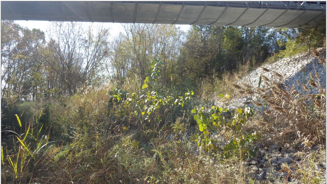
Photograph 4 – Exterior southeastern dike embankment e looking west beneath the gypsum conveyor.
