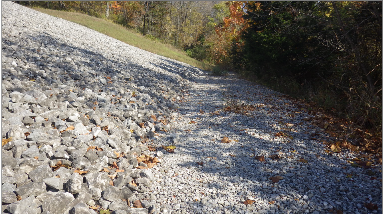
Photograph 7 – Downstream side of dam. Eastern side, looking east.
