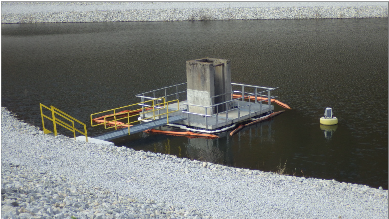
Photograph 8 – Outfall structure at southwestern corner of the LVWTS.
