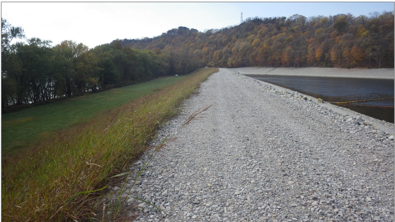
Photograph 2 – Exterior southwest dike embankment crest, looking west.
