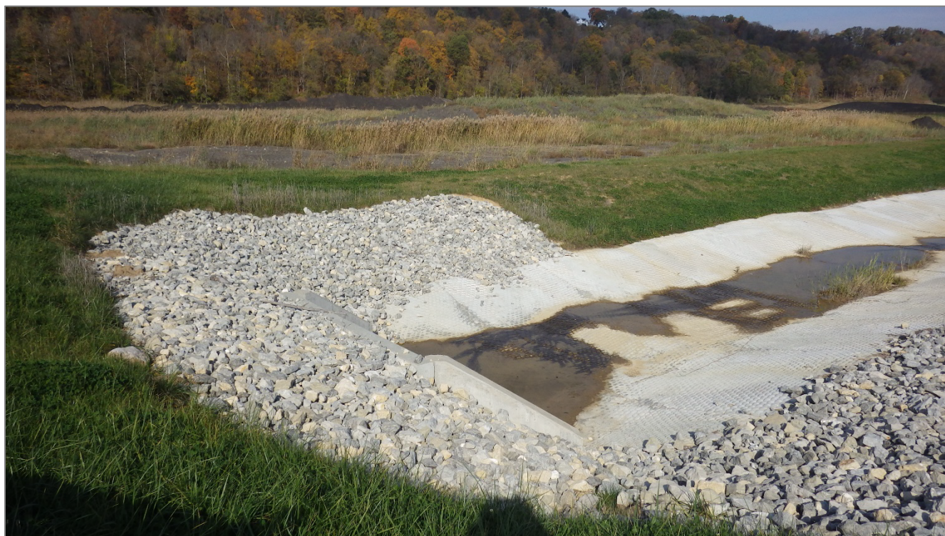
Photograph 10 – Upstream side of dam at 12 ft. x 4 ft. culvert.
