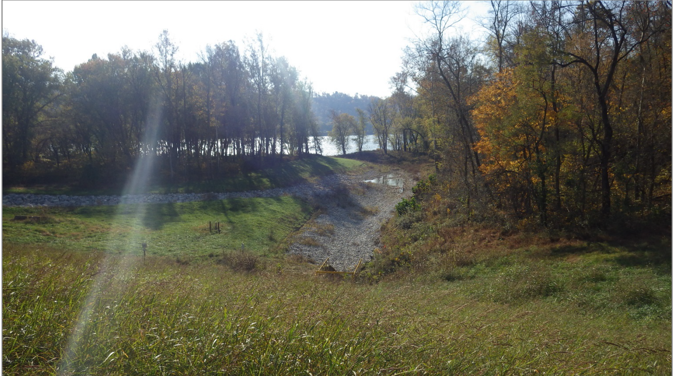
Photograph 3 – Downstream side of dam, outfall channel to the Ohio River.
