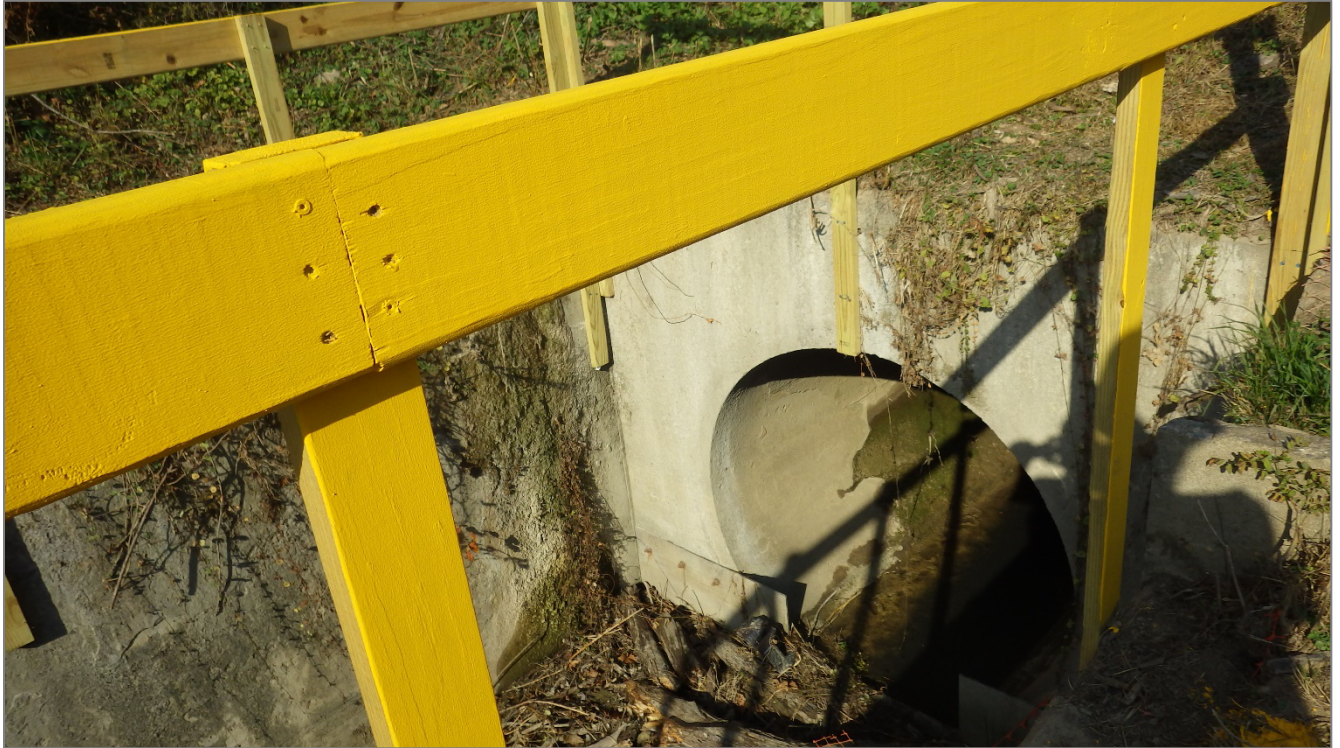
Photograph 5 – Outfall 001 outlet structure at toe of dam.
