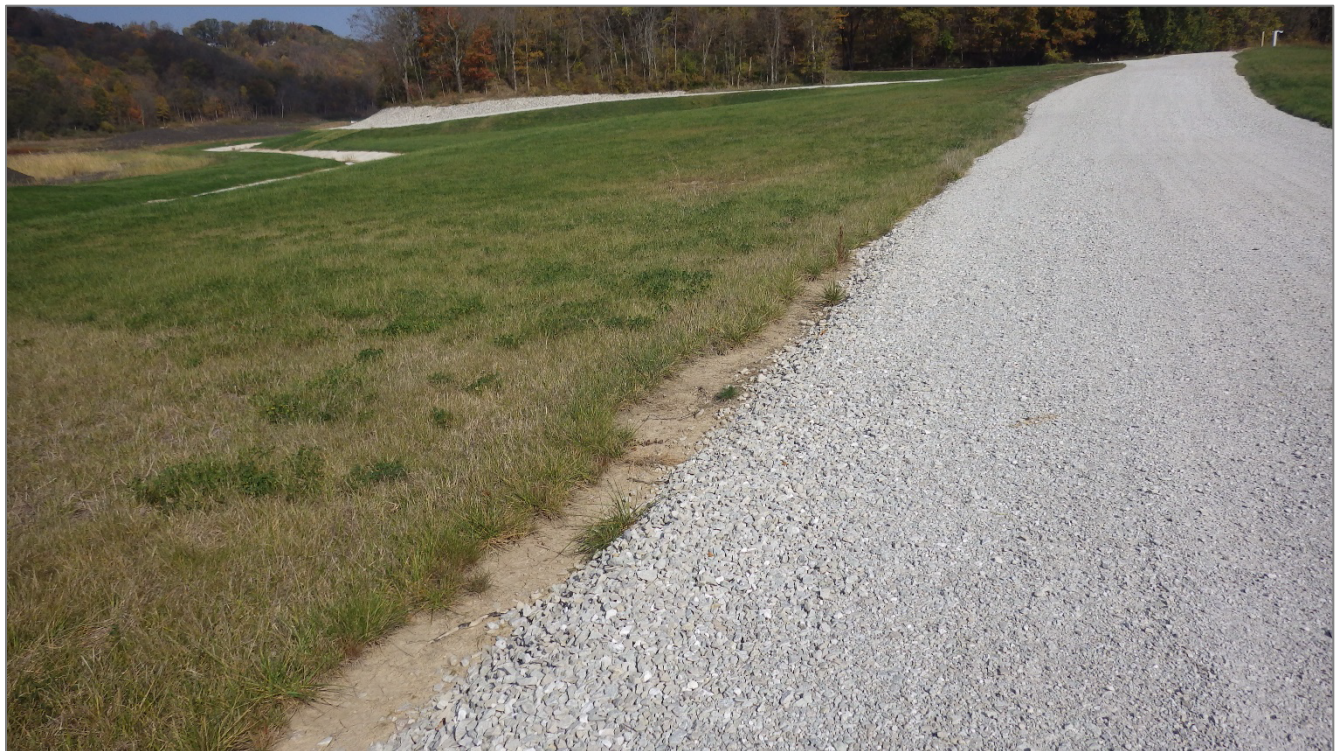
Photograph 8 – Crest of dam at the east end, looking north at access road and Phase 1 closure area.
