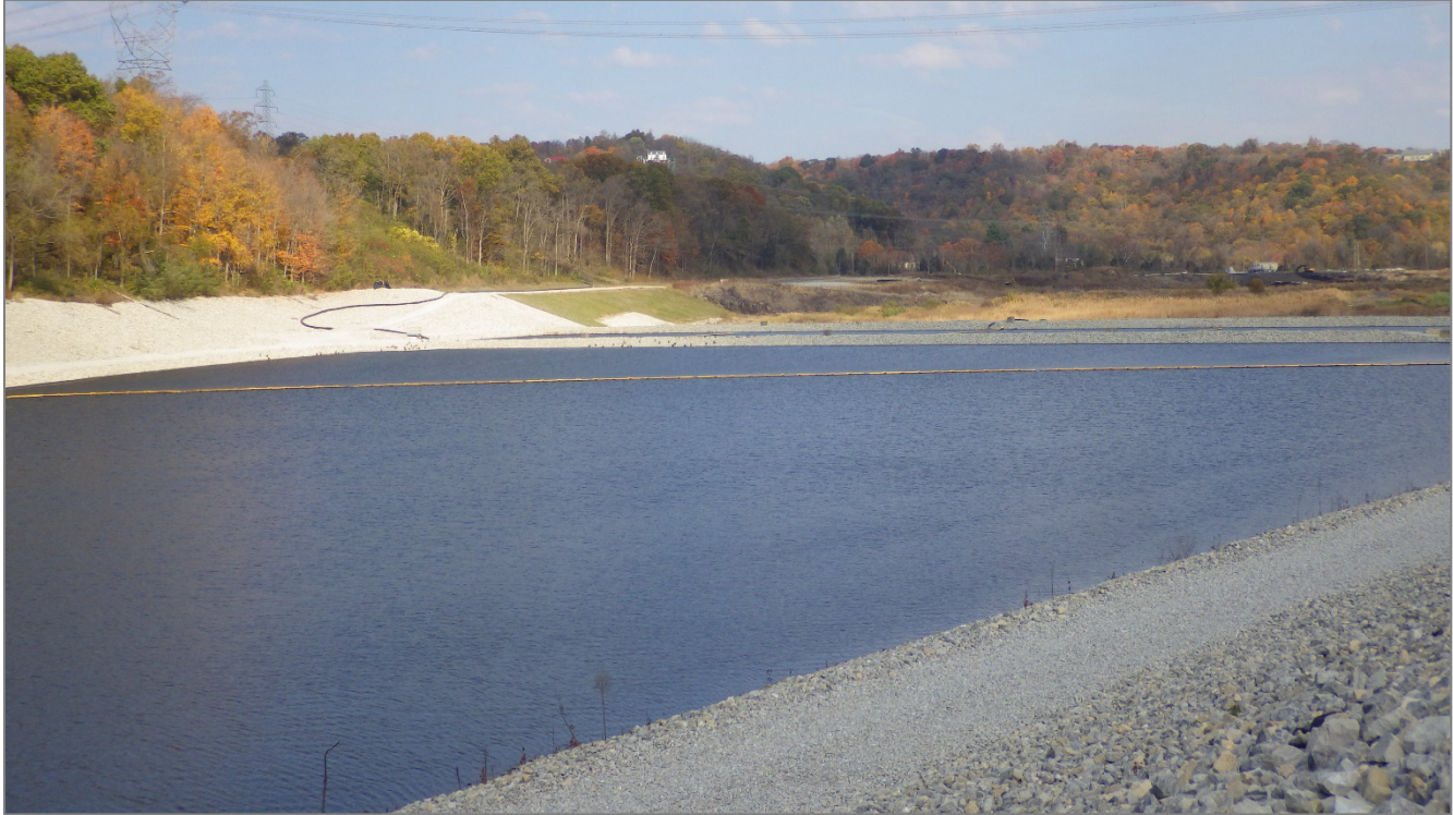
Photograph 7 – Looking north and west across LVWTS from the southern dike embankment.
