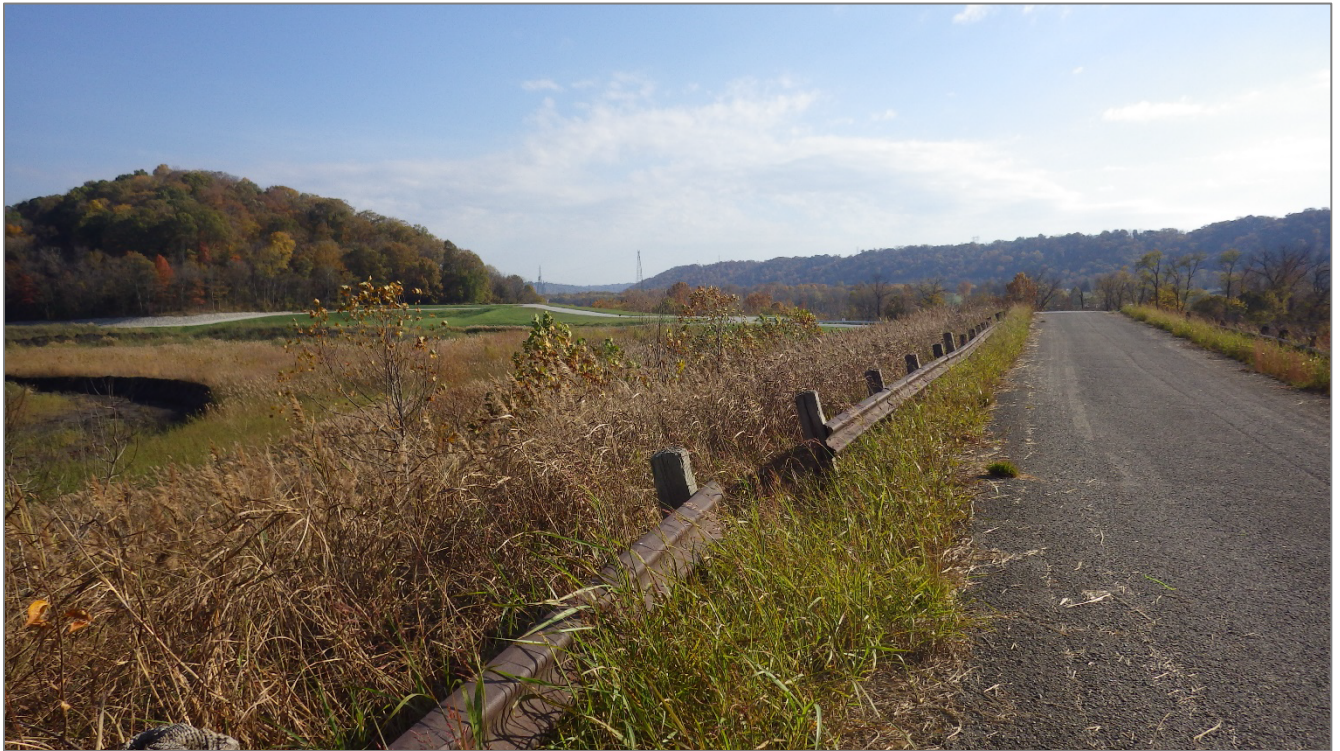
Photograph 2 – West upstream side of LRCP looking east.
