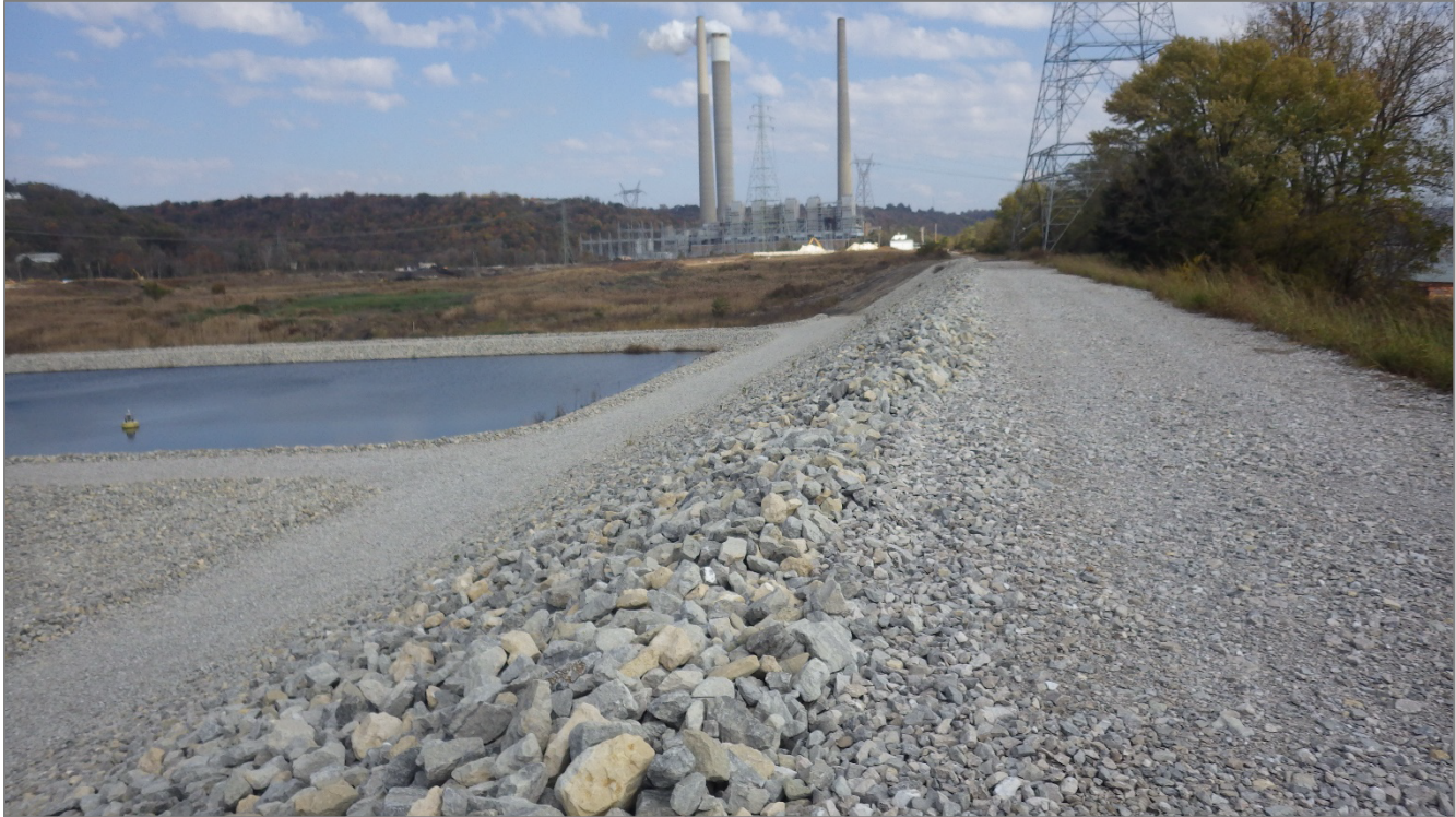
Photograph 1 – South dike embankment, upstream side looking east. LVWTS on left.
